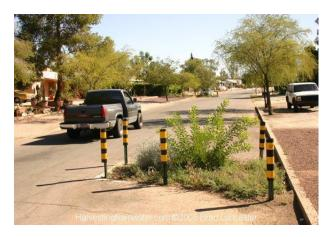
Chicanes or pull-outs with flush curbs, Midtown neighborhood, Tucson. Used where road is crowned or raised in the center, with runoff to street-side curb. Flush curb allows runoff to infiltrate soil of planting area, while surplus runoff can continue down the street. These pull-outs calm traffic by forcing it to meander. Speed humps in the area constricted by pull-outs could calm traffic even more if needed.
