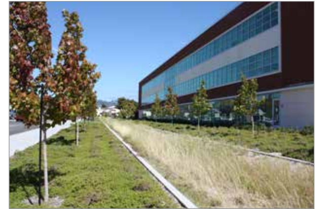
Bioswales were constructed around Civic Center to remove sediment from surface runoff water.
